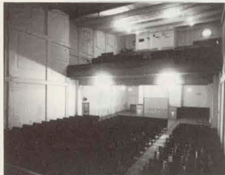
The interior of the Regent Theatre as it was being converted into the Govett-Brewster Art Gallery in 1967.
